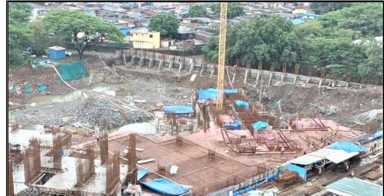
Tower B – Basement Slab & Foundation Work in Progress
